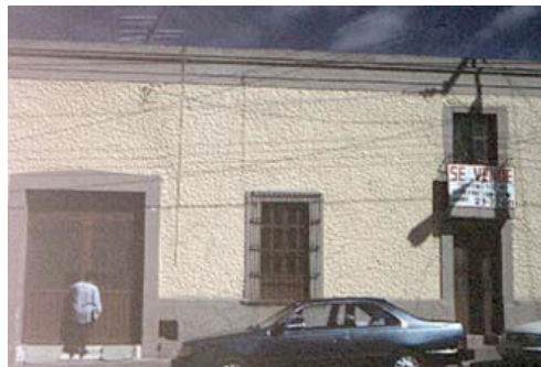
figure 09. Example of catalogued building with a door turned into a window
